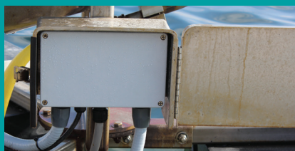
Water shield covering junction box to provide dual protection for water ingress to electrical terminations
