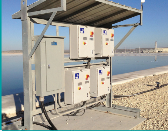
Galvanized control panel shelter with load center and machine control panels
